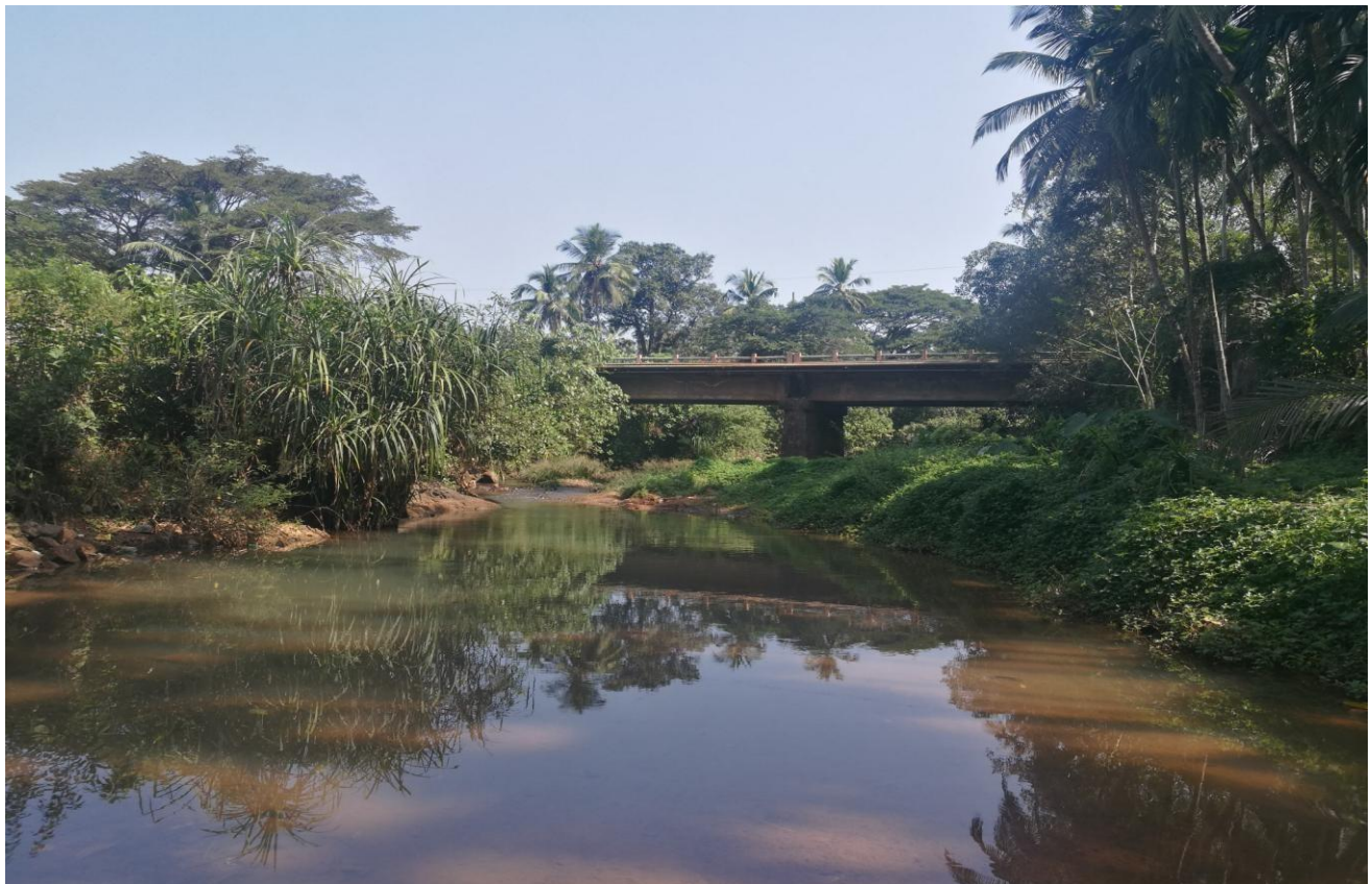
Fig 1: Mogral river at Edneer bridge
